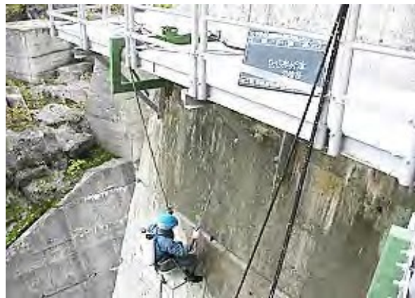
At a downstream side of a dam body: Spraying CS-21
