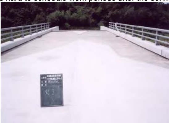
Waterproofing of floor slabs of a road bridge
