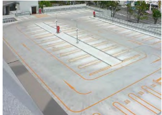
Waterproofing of a multilevel parking tower
