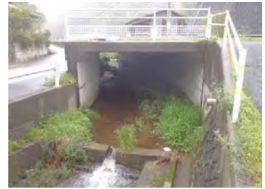
Surface protection of a box culvert
