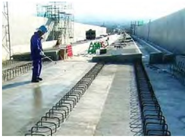
Waterproofing of floor slabs
