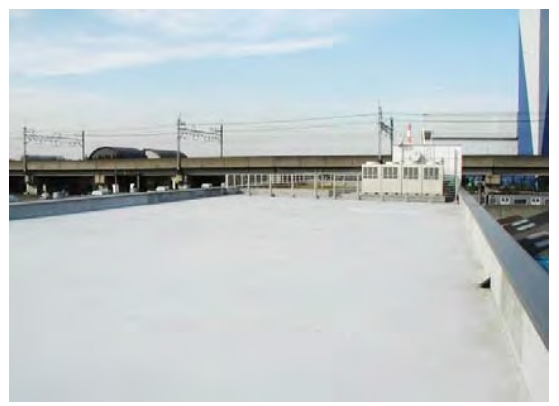
Waterproofing of a roof
