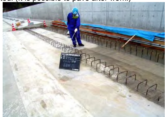
Waterproofing of floor slabs of a railway bridge
