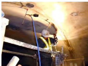
High-pressure injection for crack repair
