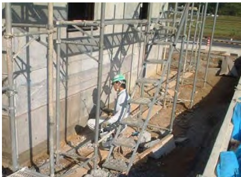
Exterior waterproofing of a basement
