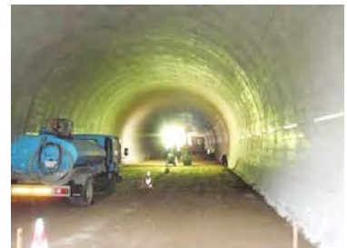
Surface protection of a tunnel lining
