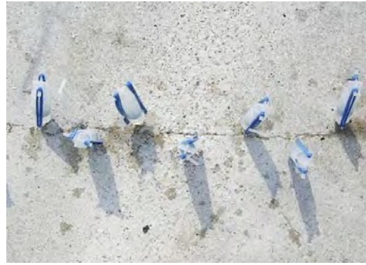
Water leakage repair at a floor slab: CS Plug
