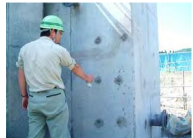
Treatment of imprinted holes for separator end
