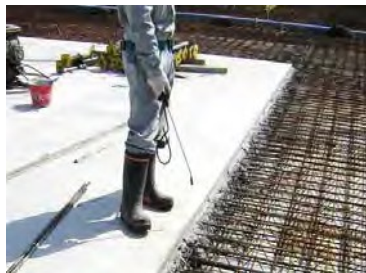
Treatment of placing joints (Vertical joints)
