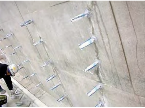
Crack repair at a bridge footing: Injection plug
