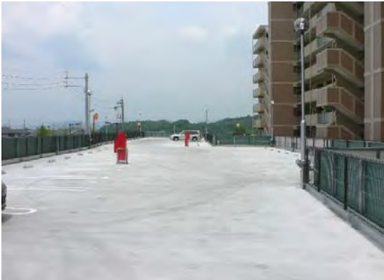
Waterproofing of a multilevel parking tower
