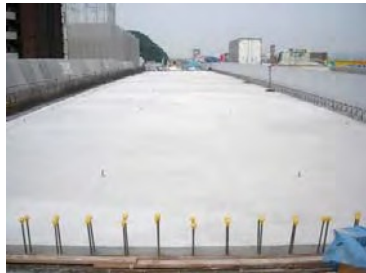
Surface protection of floor slabs
