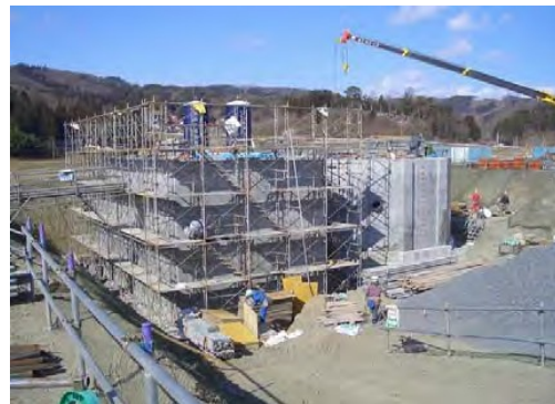
Waterproofing of a water tank
