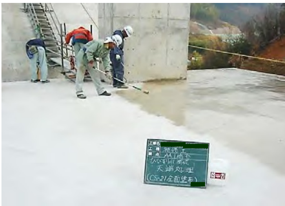
On an abutment: Spreading CS-21
