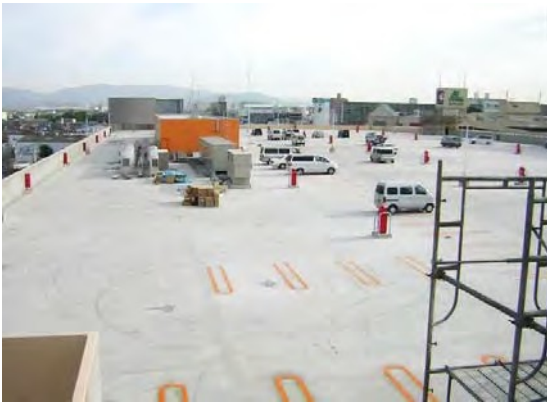
Waterproofing of a parking lot on the roof
